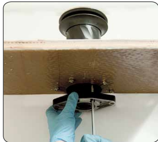
2. Tighten the six screws ( \approx 8 Nm/ 71 in-lb)
